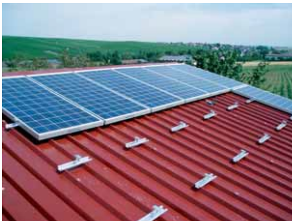
The ROOF-VENT support profiles are only riveted to the roof at the points required by the module installation.
