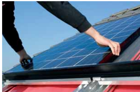
Simple insertion of the modules
